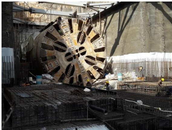
Figure 1. EPB machine used in the Tabriz city metro line 2 project [31]
