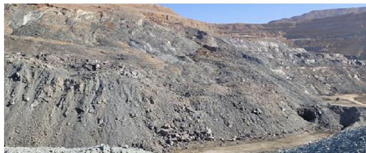
Fig. 15. A view of the failure that happened on the north wall of mine No. 4.
