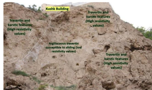
Fig. 12. Representation of the Geology Downstream of the Koshk Structure and Its Geoelectrical Interpretation.
